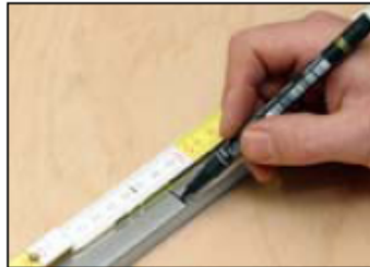
Measure and mark the aluminium section to door size only at end with round actuator (for double actuation models only)
