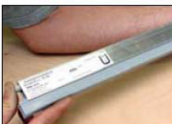
Test operation of seal by pushing actuator at both ends
