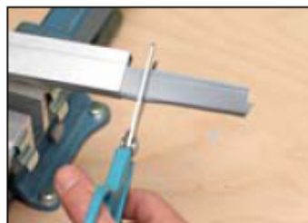
Cut seal profile with sharp knife or scissors allowing an extra 3 - 5mm for gap between door and frame
